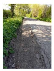
Damage from traffic to verge on Five Oak Lane close to Winery, causing ditches to be eroded and collapse
